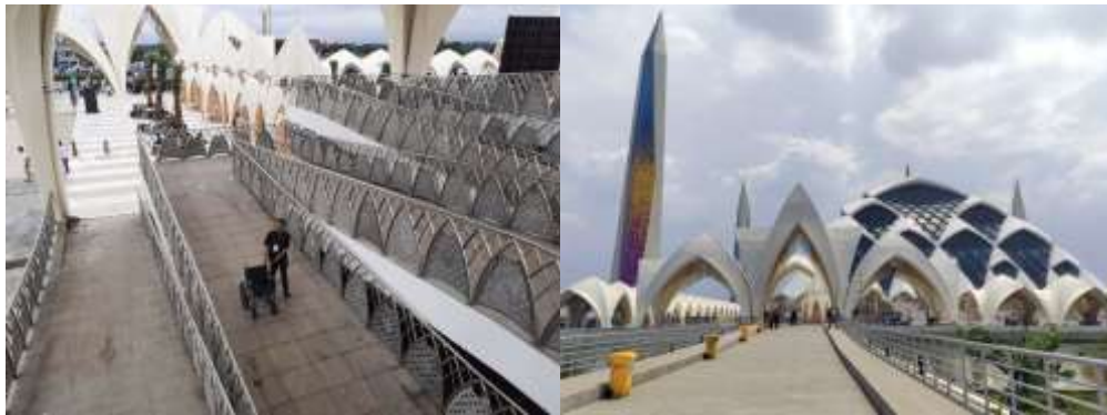
Figure 8. Ramp (inclusive zone)
